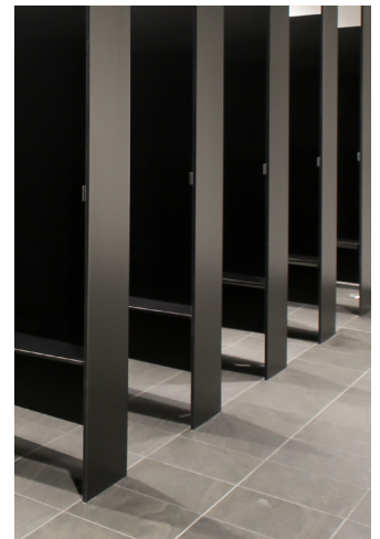
Concealed Fixed Panels Mounted Directly to the Floor
