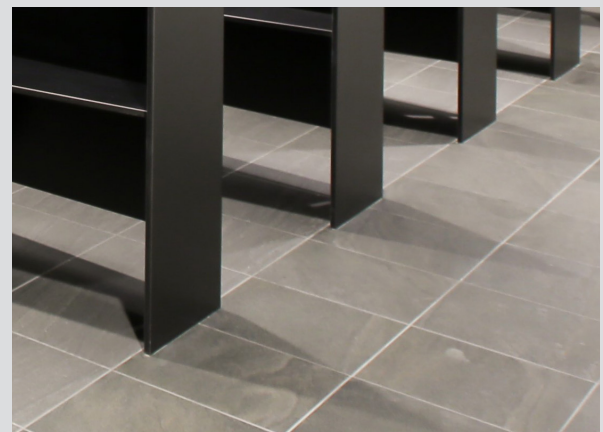
Concealed Fixed Panels Mounted Directly to the Floor
