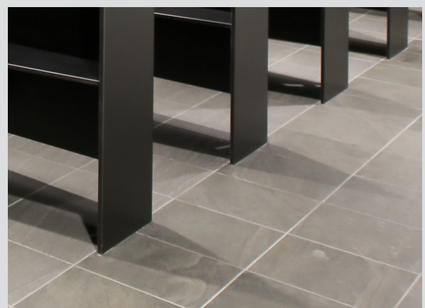
Concealed Fixed Panels Mounted Directly to the Floor
